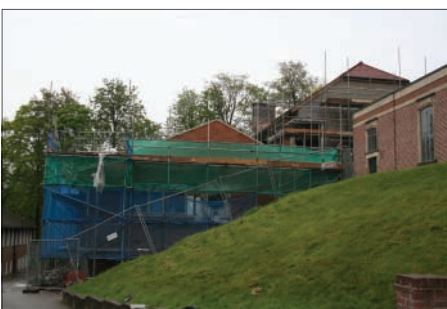
New Science Block in progress
